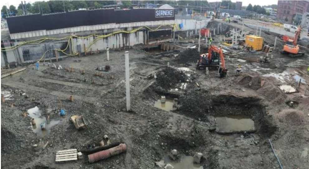
Figure 7 A view of the construction phase
