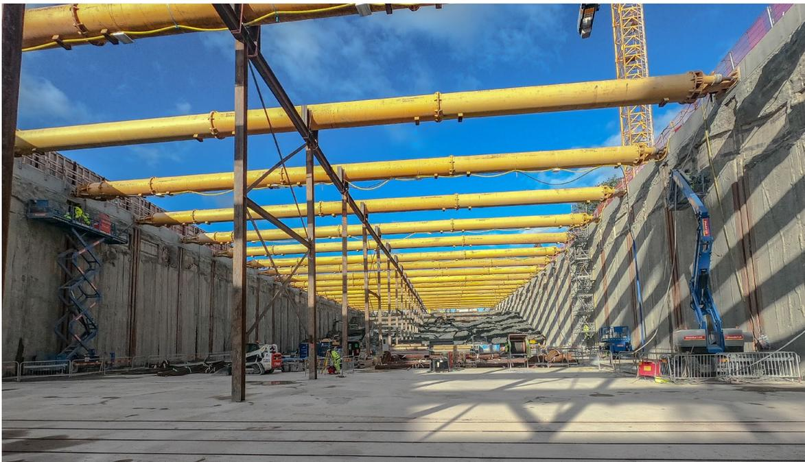
*Figure 1. View into the already excavated construction pit shows the D-Walls and and the enormous free space to construct the cut and cover tunnel.*
