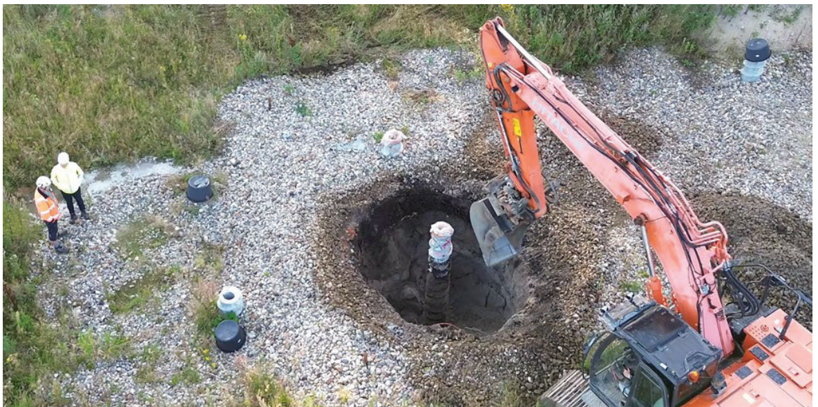
Fig. 6. Extraction of concrete screw pile after installation and static load test
