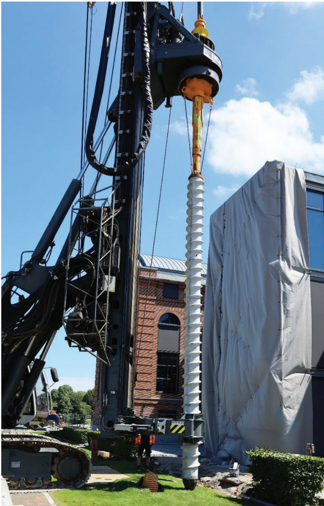
Fig. 13 Installation of CPSP directly up against existing structures.
