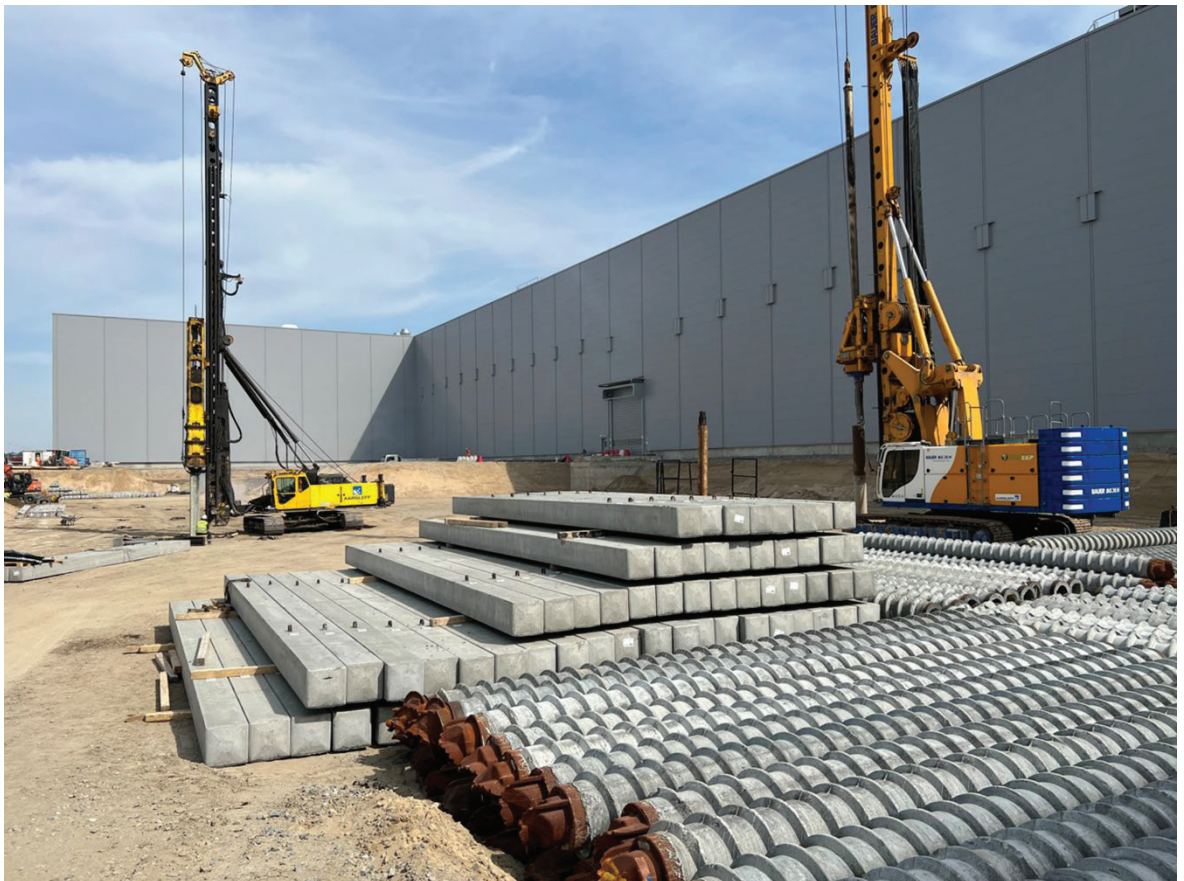
Fig. 9 Piling at EV Gigafactory near Berlin, Germany
