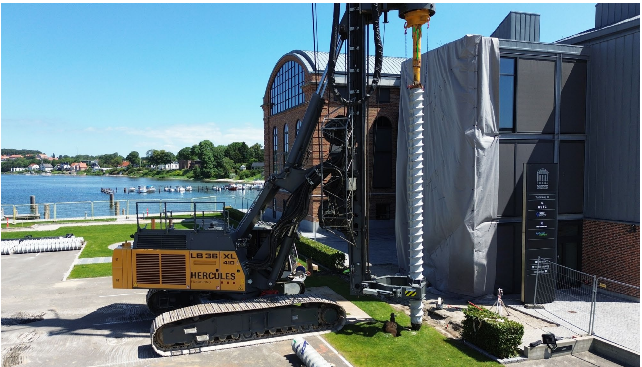
Fig. 1 -Installation of Prefab Screw Pile
