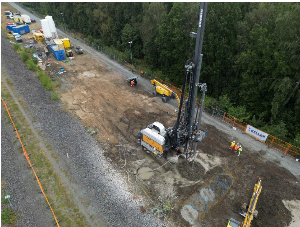
Figure 8 Drone picture showing test field with WDM
